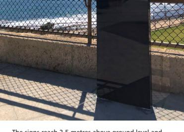
The signs reach 2.5 metres above ground level and are well anchored on a concrete support base. An inner frame is covered by an aluminium exterior which has been 2 pac painted to withstand the harsh coastal conditions.
